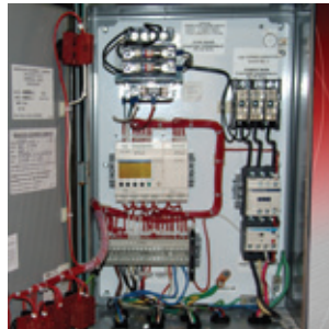
Front opening control panel eliminates the need for 48" side clearance as required by NEC® standards.
